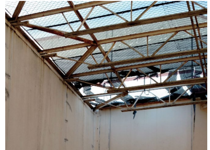
Damage in lightwell at Satellite Corrections facility.
