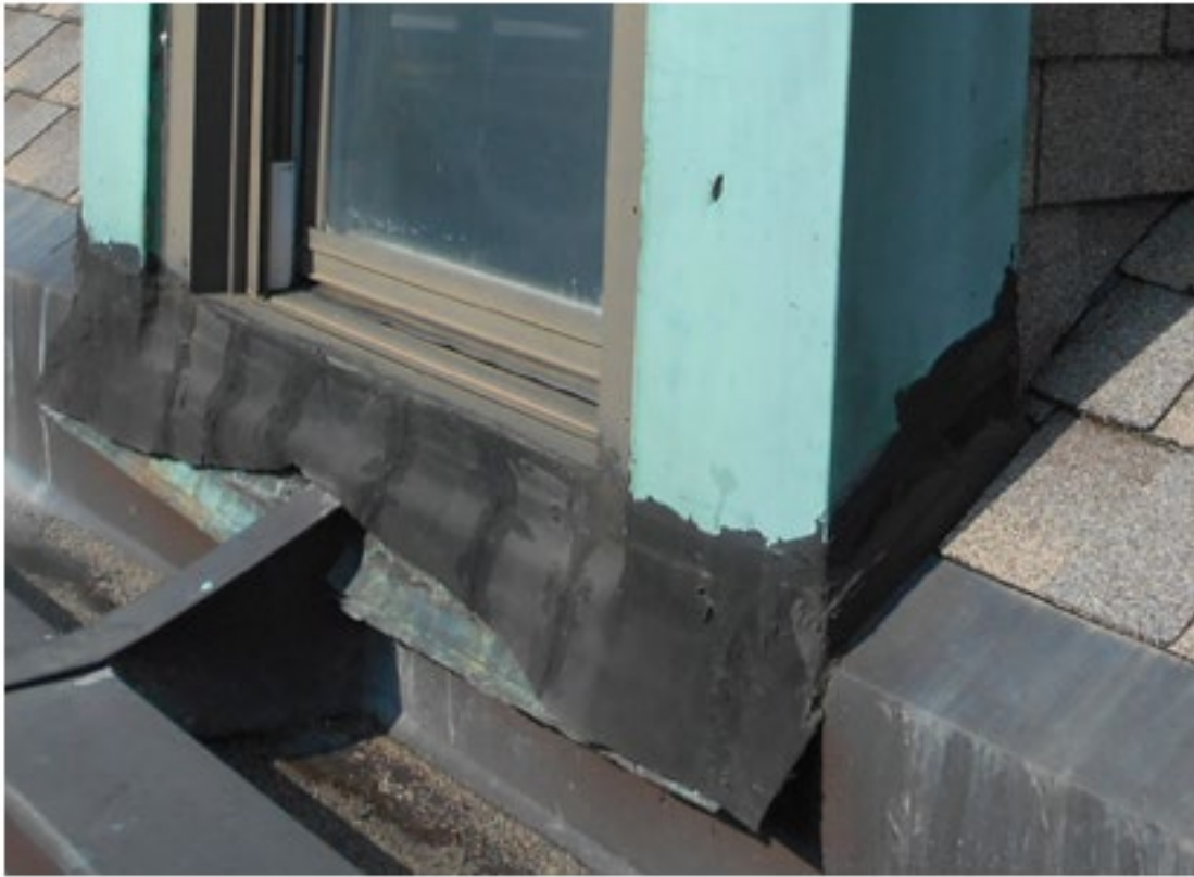
Flashing repairs needed around courthouse windows.
