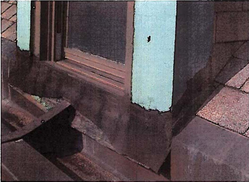
*Flashing repairs needed around courthouse windows.*
