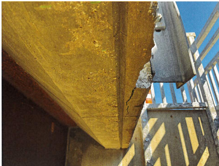
Spall and cracking under post two - approximately 5' compromised
