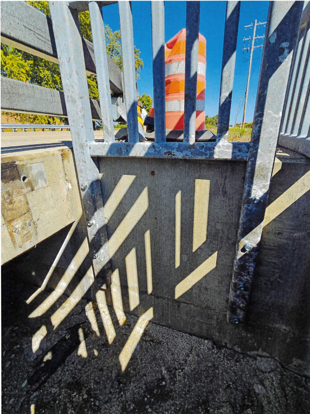
Railing between bridge and pedestrian bridge – has been re-bolted in and is secure.
