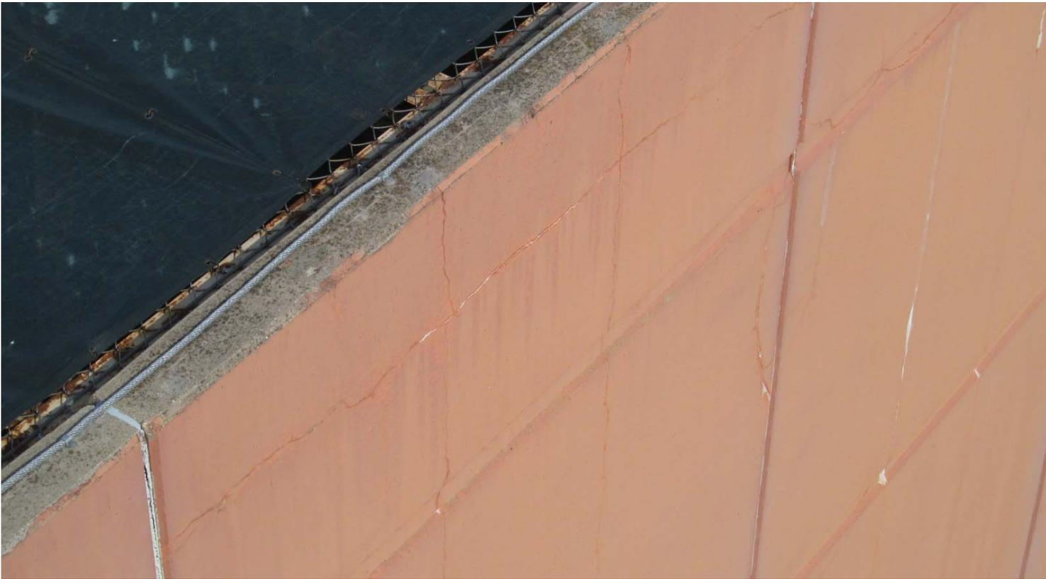
**Photograph #24: East Exercise Yard Wall Cracking**
