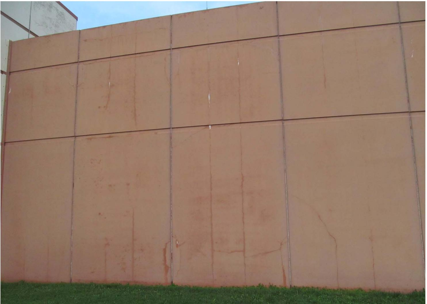
Photograph #21: East Wall Cracking Pattern
