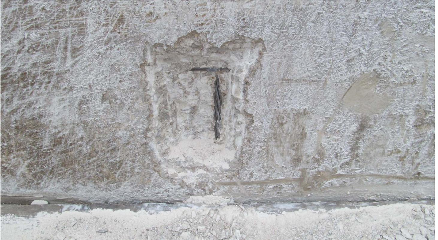
**Photograph #12: The left-center prestressing strand was corrosion free.**
