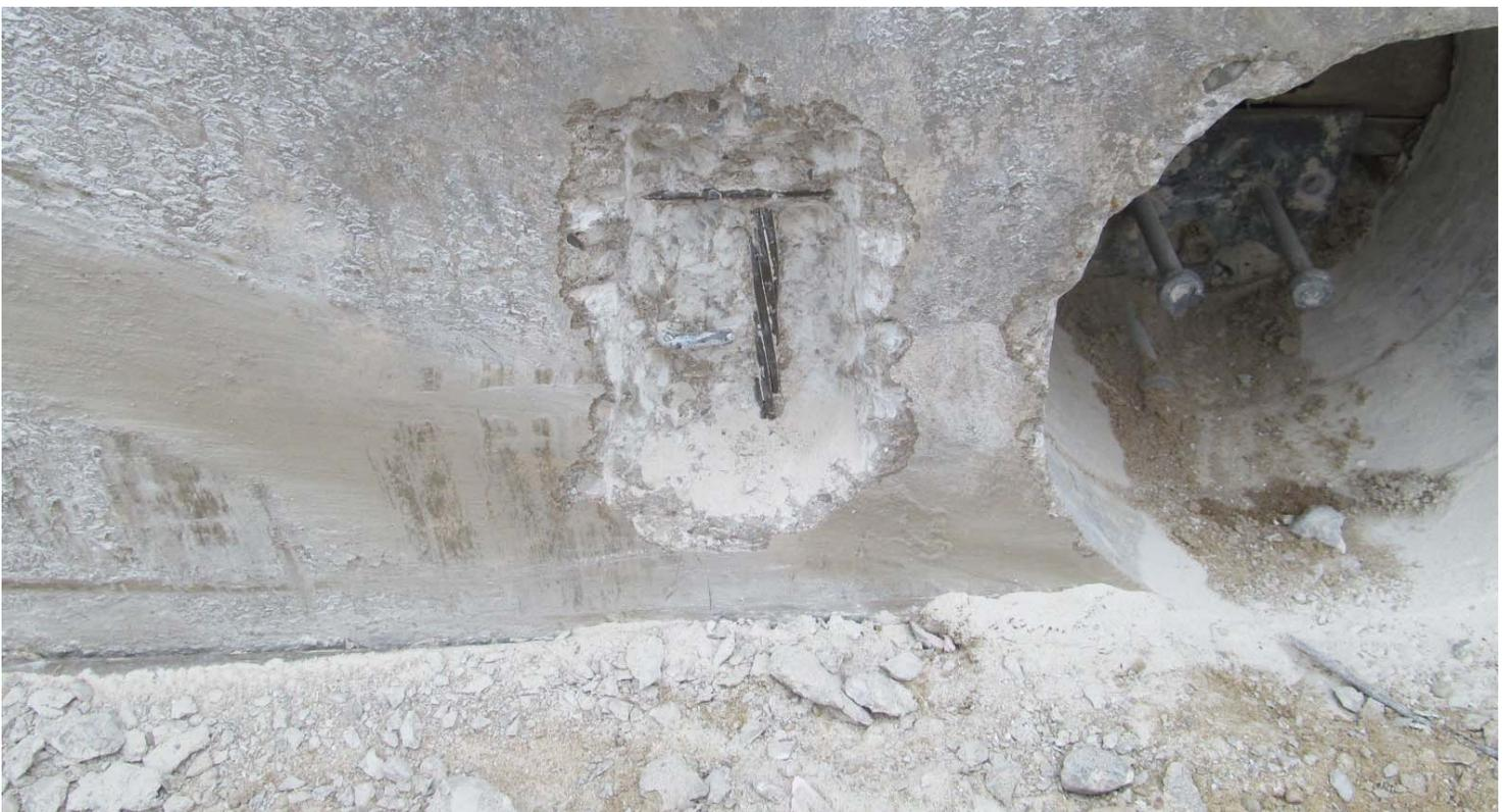
**Photograph #13: The right-center prestressing strand was corrosion free.** 21
