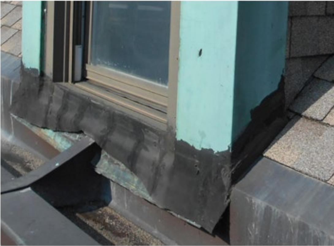
*Flashing repairs needed around courthouse windows.*
