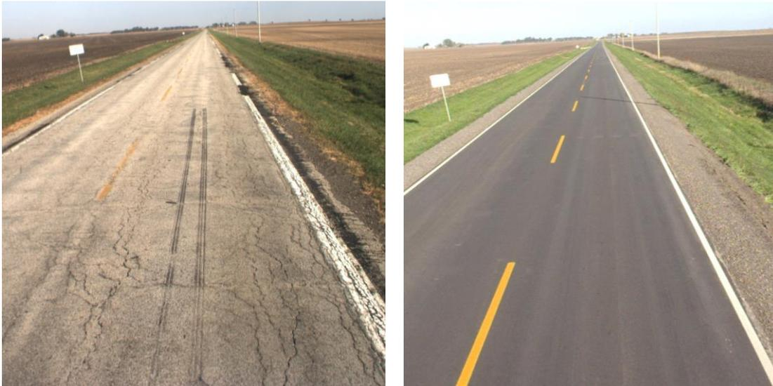
Figure 1. Champaign County's PMS optimizes the expenditure of construction funds over the long-term by choosing the most appropriate treatment and timing for road improvements (County Highway 23, pre- and post-2017 construction).
