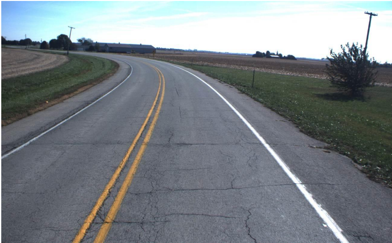
Figure 2. Digital images taken every 20 feet show pavement distresses and roadside assets.
