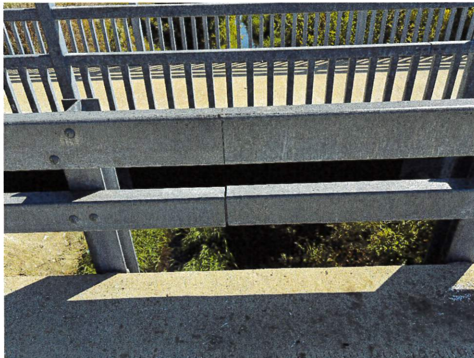
SM Rail Splice between Post 7 (left) and Post 8 (right).
