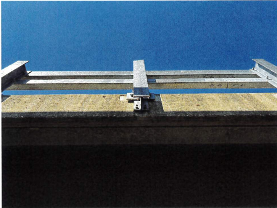
Post 8 (center) twisted – can also see SM rail splice to right of post 8
