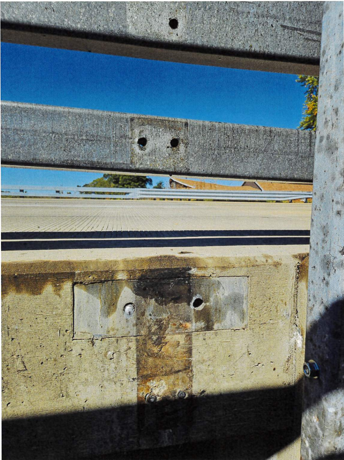
Post One – Post obliterated and Bolts missing or sheared
