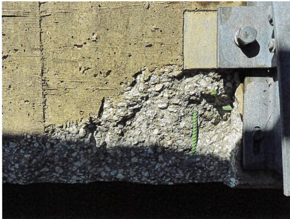
Post two – spall – epoxy coated rebar in decent shape.
