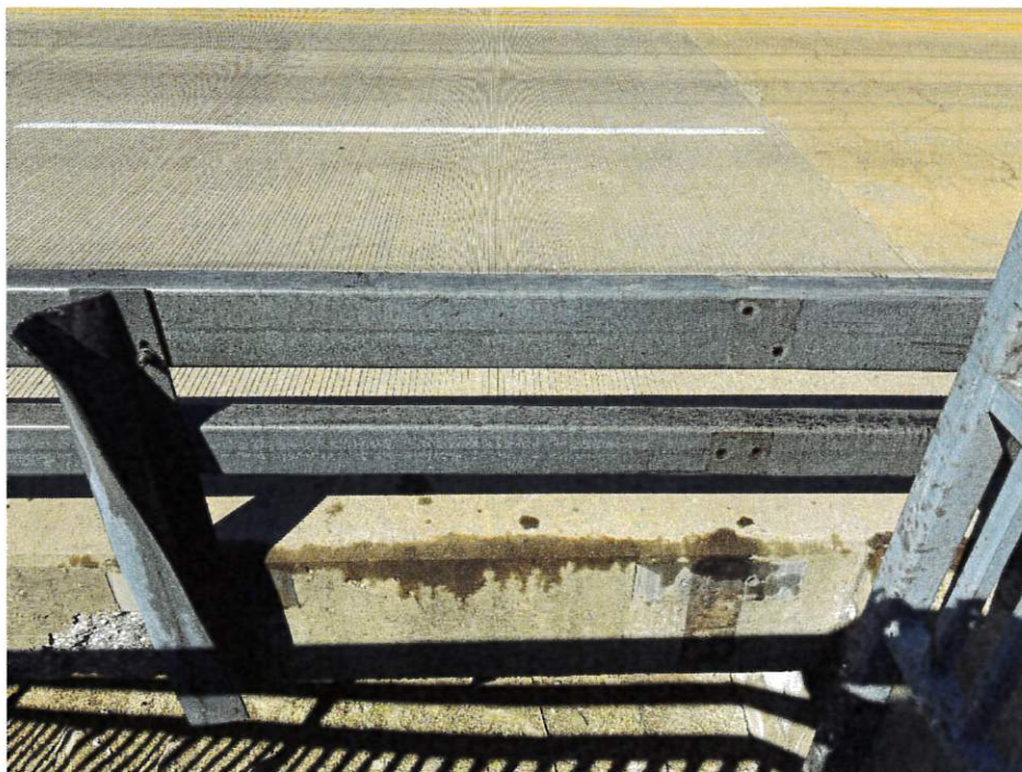
Post one (missing) and Post two (twisted) from north east corner
