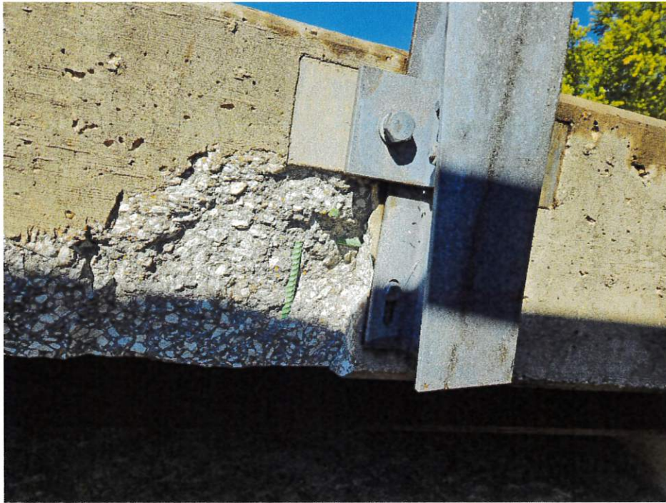
Post two spall south of post (3'-3" x 13" triangular)
