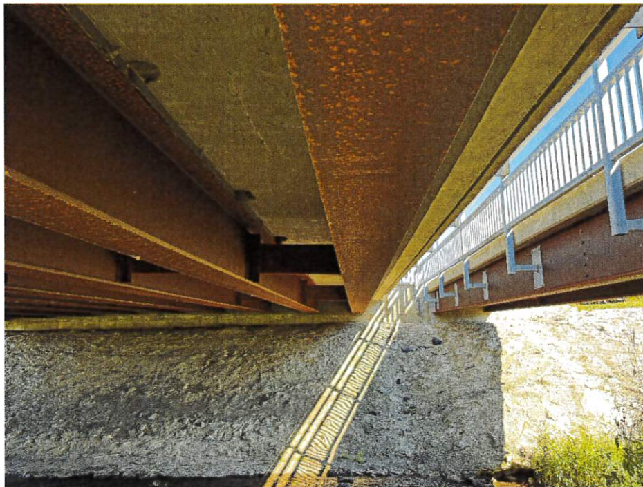
Looking North at East beam – No deficiencies noted.
