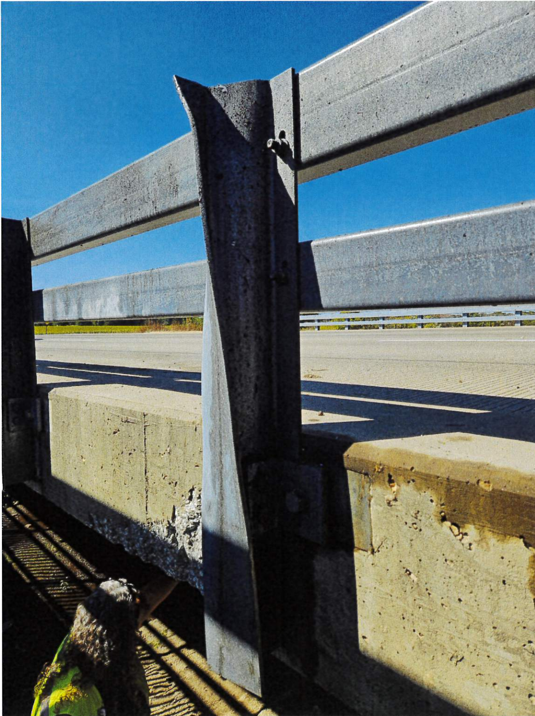
Post two twisted, and spall visible
