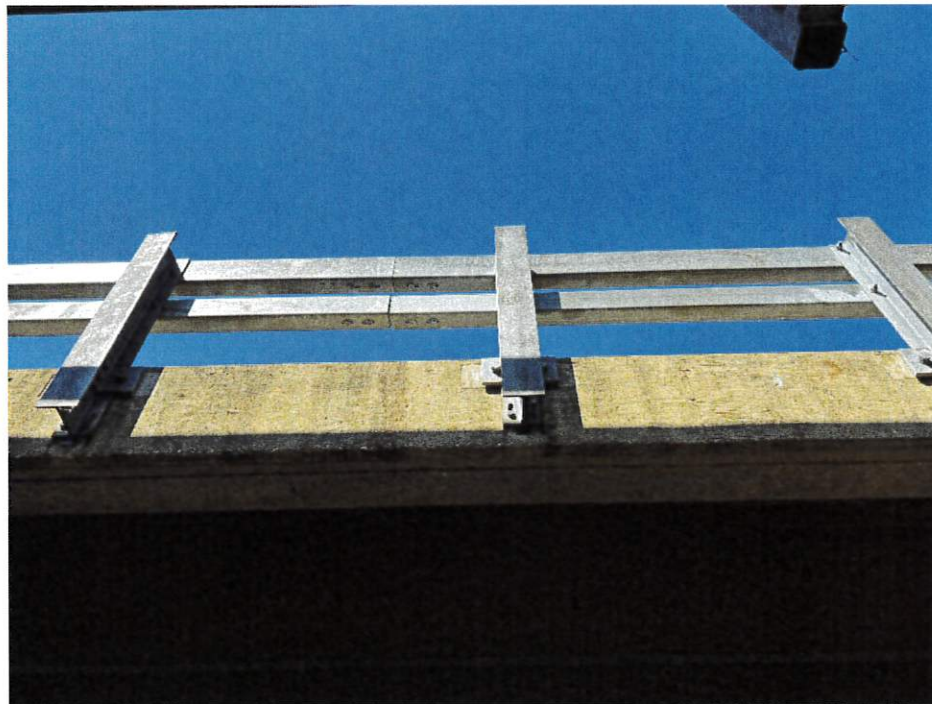
Posts 8, 7, 6 from left in photo. Also visible the SM rail splice between 8 and 7.
