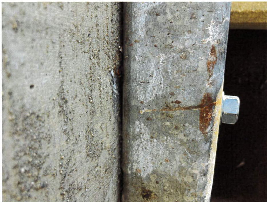
New bolt at railing between bridge and pedestrian bridge – north side – concrete spall behind railing. Typical both pictures on page.
