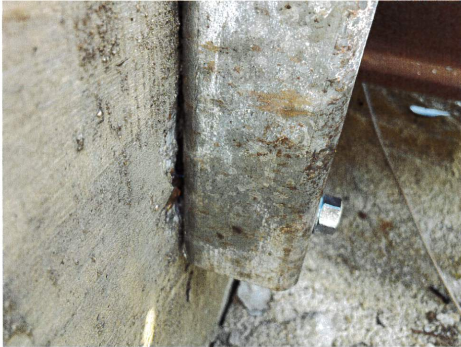
New bolt at railing between bridge and pedestrian bridge – north side – concrete spall behind railing. Typical both pictures on page.
