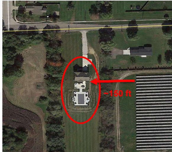
Dominion Indy III Solar Farm October 2016
