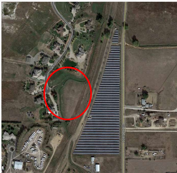
Brighton PV Solar, Adams County, CO June 2016
