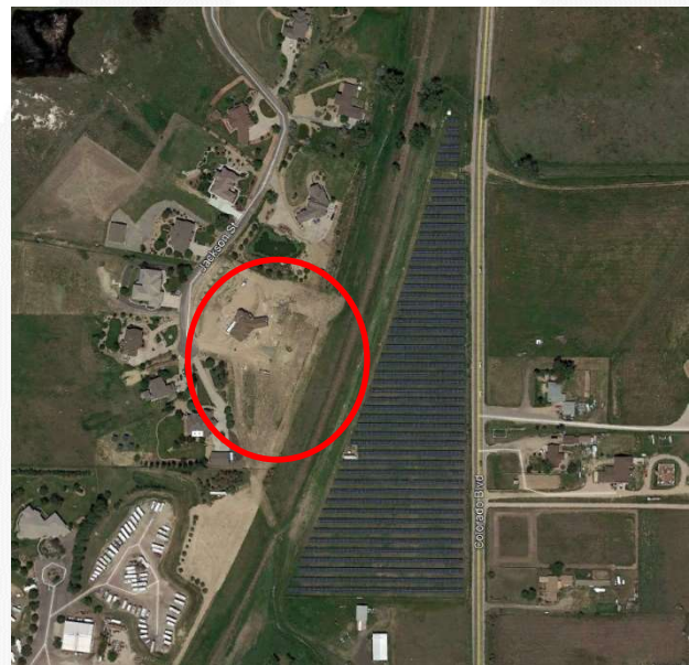
Brighton PV Solar, Adams County, CO June 2017
