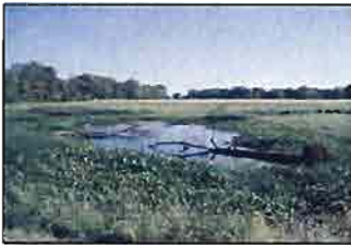
Stormwater Wetland Engineering APWA Project of the Year Award and ACEC Engineering Excellence Merit Award
