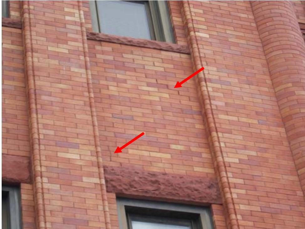
**Photo No. 1:** West façade spandrel area – typical area of step cracking with cracked brick and open mortar joints.
