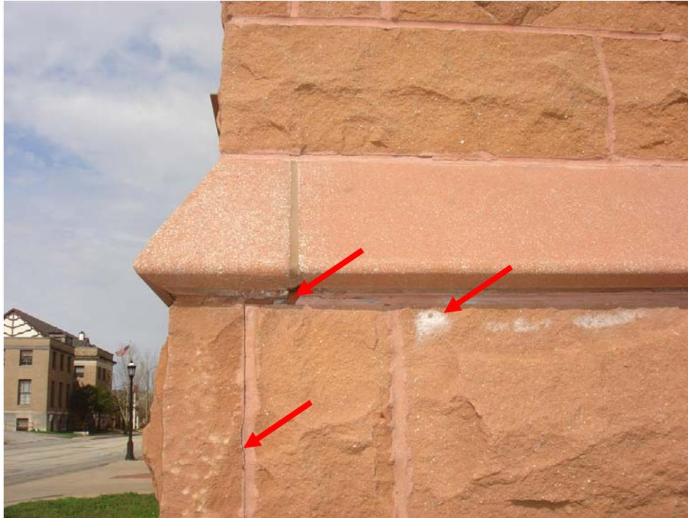
**Photo No. 1:** North façade cast stone base and horizontal band – minor cracked and open mortar joints and efflorescence. Note: Cast stone was used on the new addition to simulate cut natural stone.
