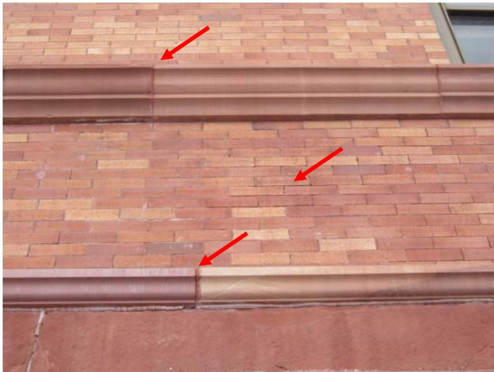
**Photo No. 2:** South façade brick spandrel and sandstone horizontal bands – typical area of open mortar joints at brick spandrel areas and occasionally cracked and open mortar joints at sandstone bands.
