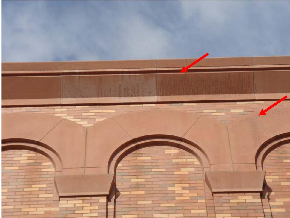
**Photo No. 3:** North façade cast stone cornice – staining.
