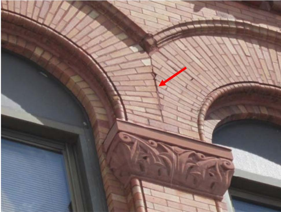
**Photo No. 3:** West façade third floor arched window head – open joints at brick masonry.
