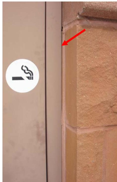
**Photo No. 5:** North façade grade level exit door – no sealant in joint between door frame and cast stone building base.
