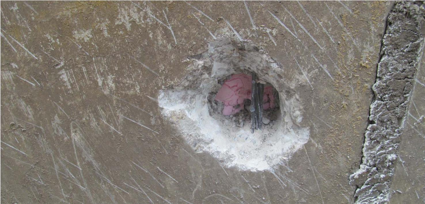
**Photograph #20: The strand on the right side of the panel was corrosion free.**
