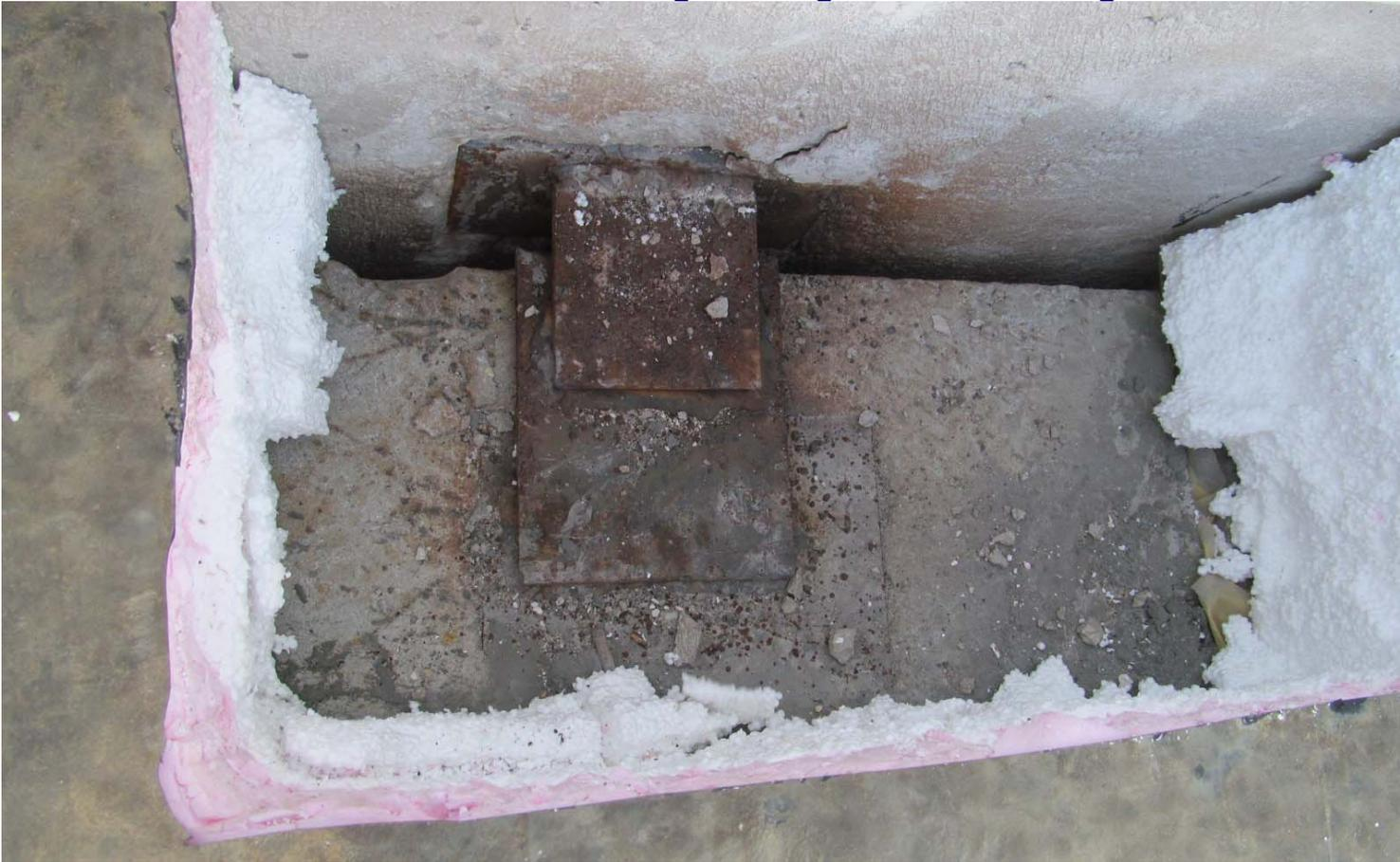
**Photograph #28: Rust on roof plank / wall panel connection, East Wall**
