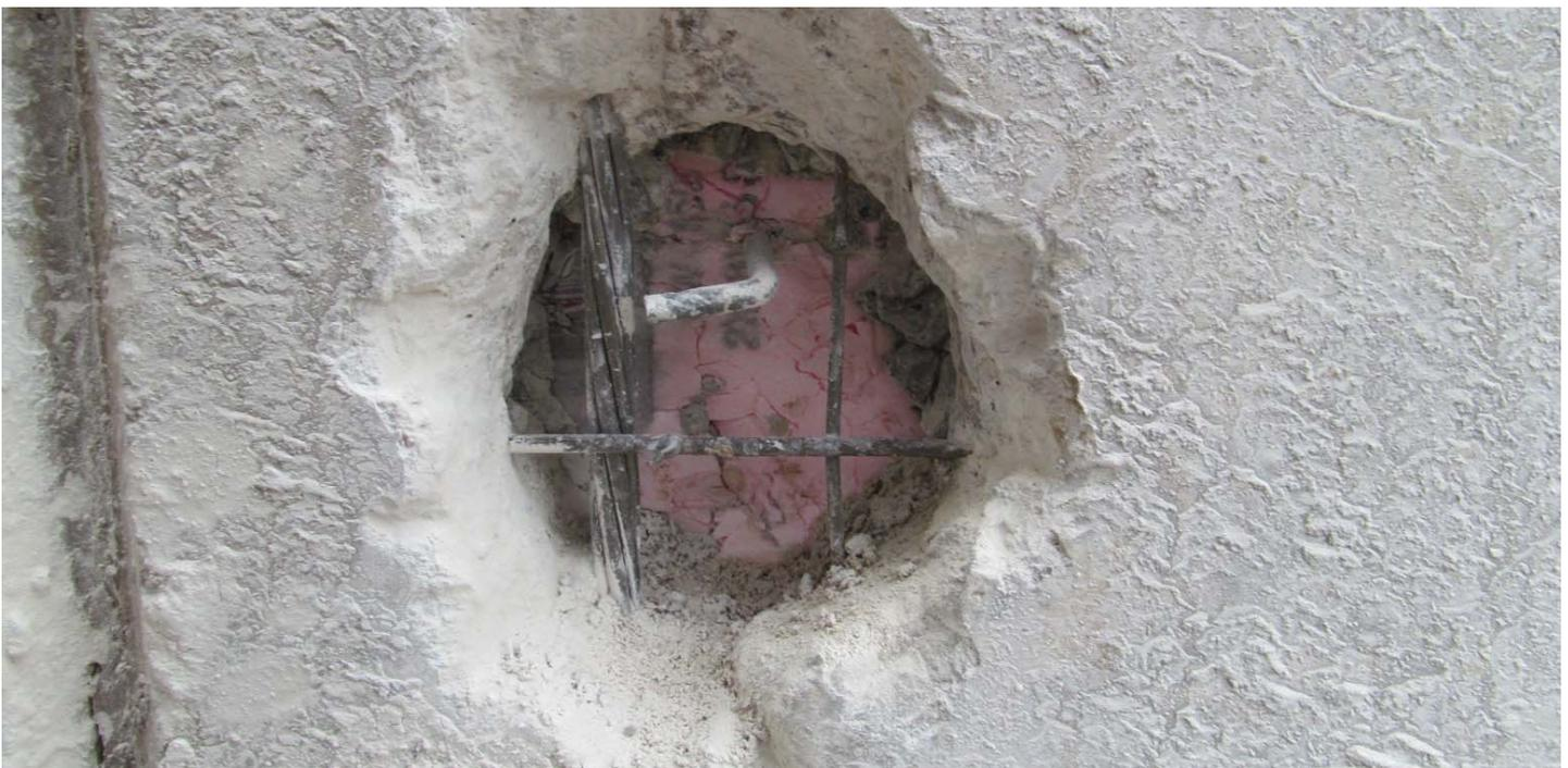
**Photograph #17: The strand on the left side of the panel was corrosion free. The L-shaped tie wire is the mechanical connection between concrete layers.**
