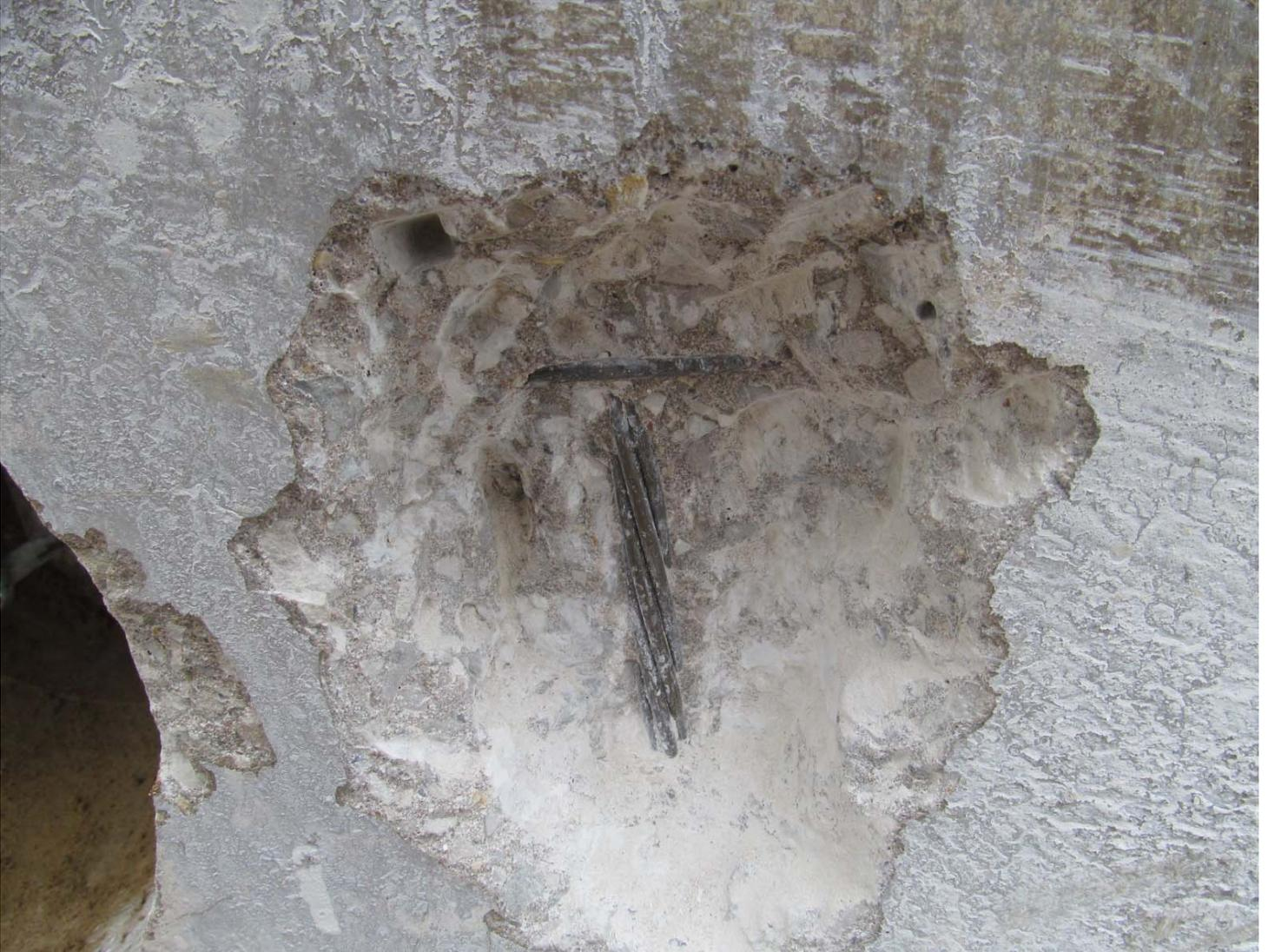
**Photograph #18: The left-center prestressing strand was corrosion free.**
