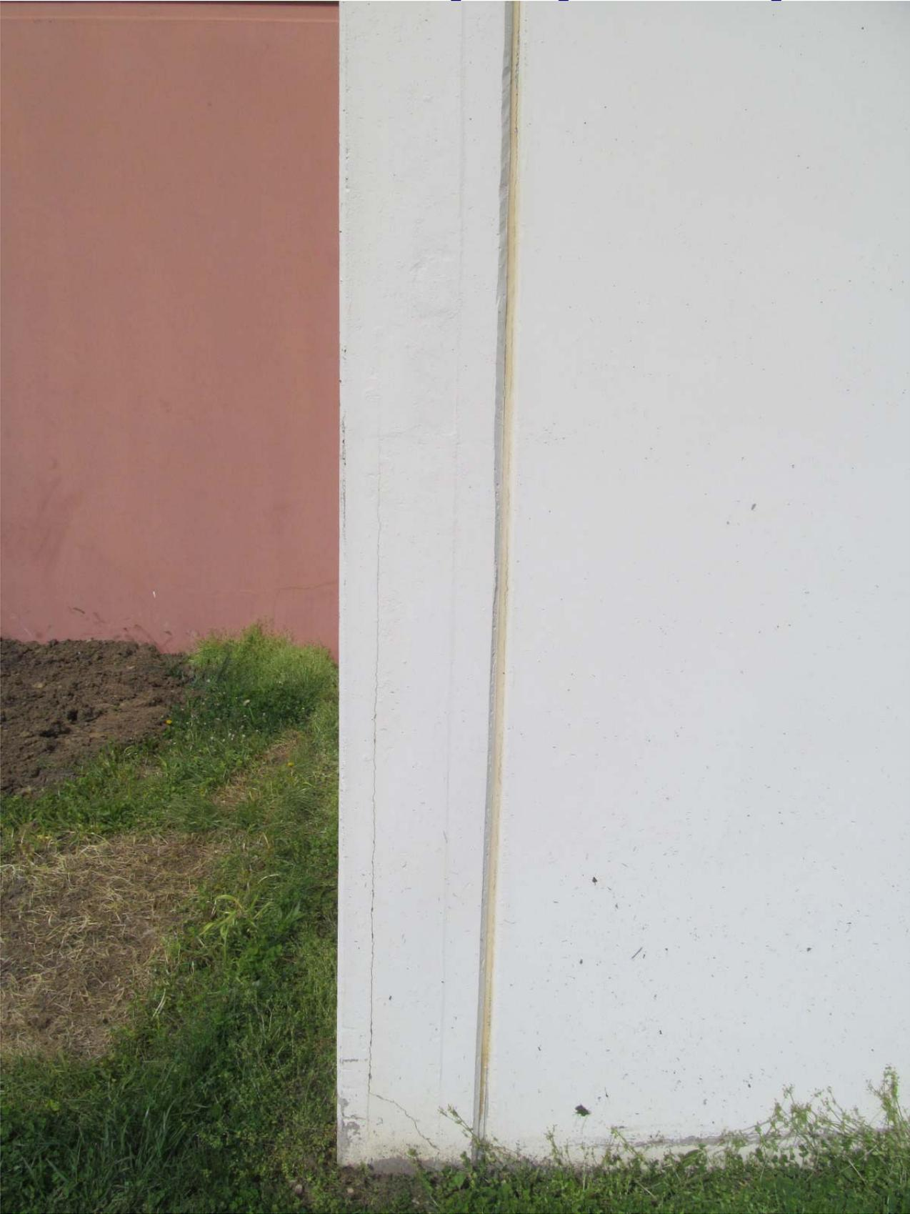
**Photograph #26: East Wall Panel Edge** The insulation was cut or held back from the Wall Panel Edge. The mortar over the insulation is cracked.
