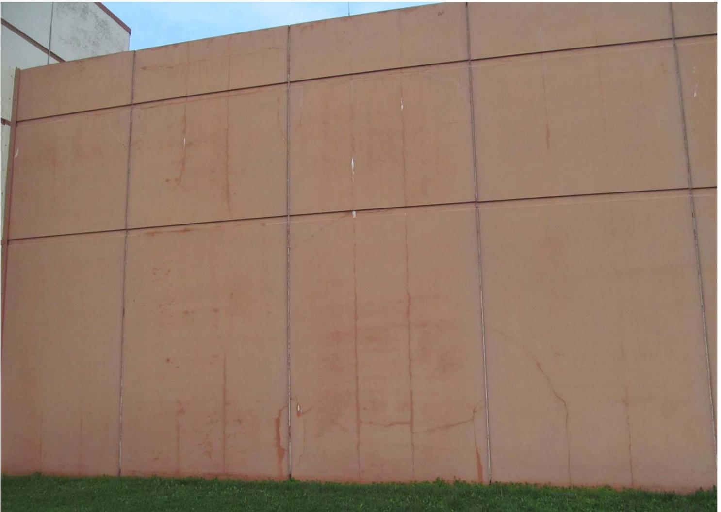
Photograph #21: East Wall Cracking Pattern
