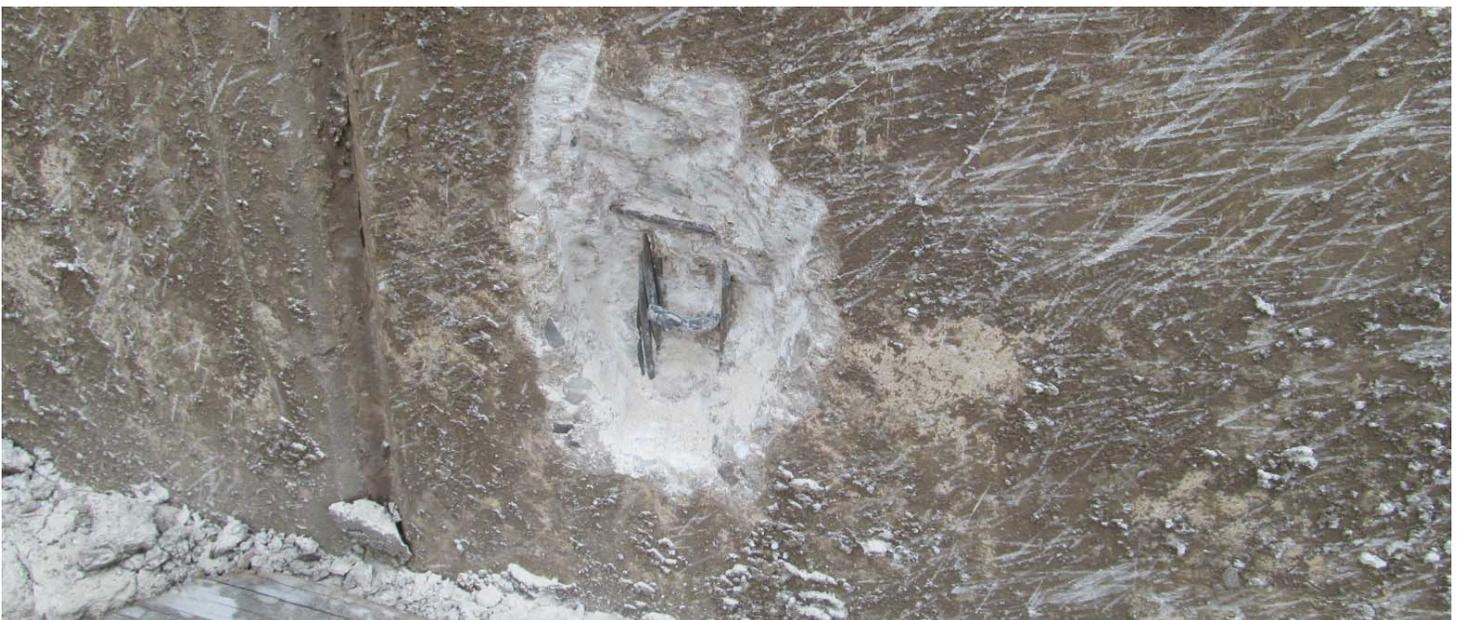
**Photograph #11: The strand on the left side of the panel was corrosion free.<sup>20</sup>**
