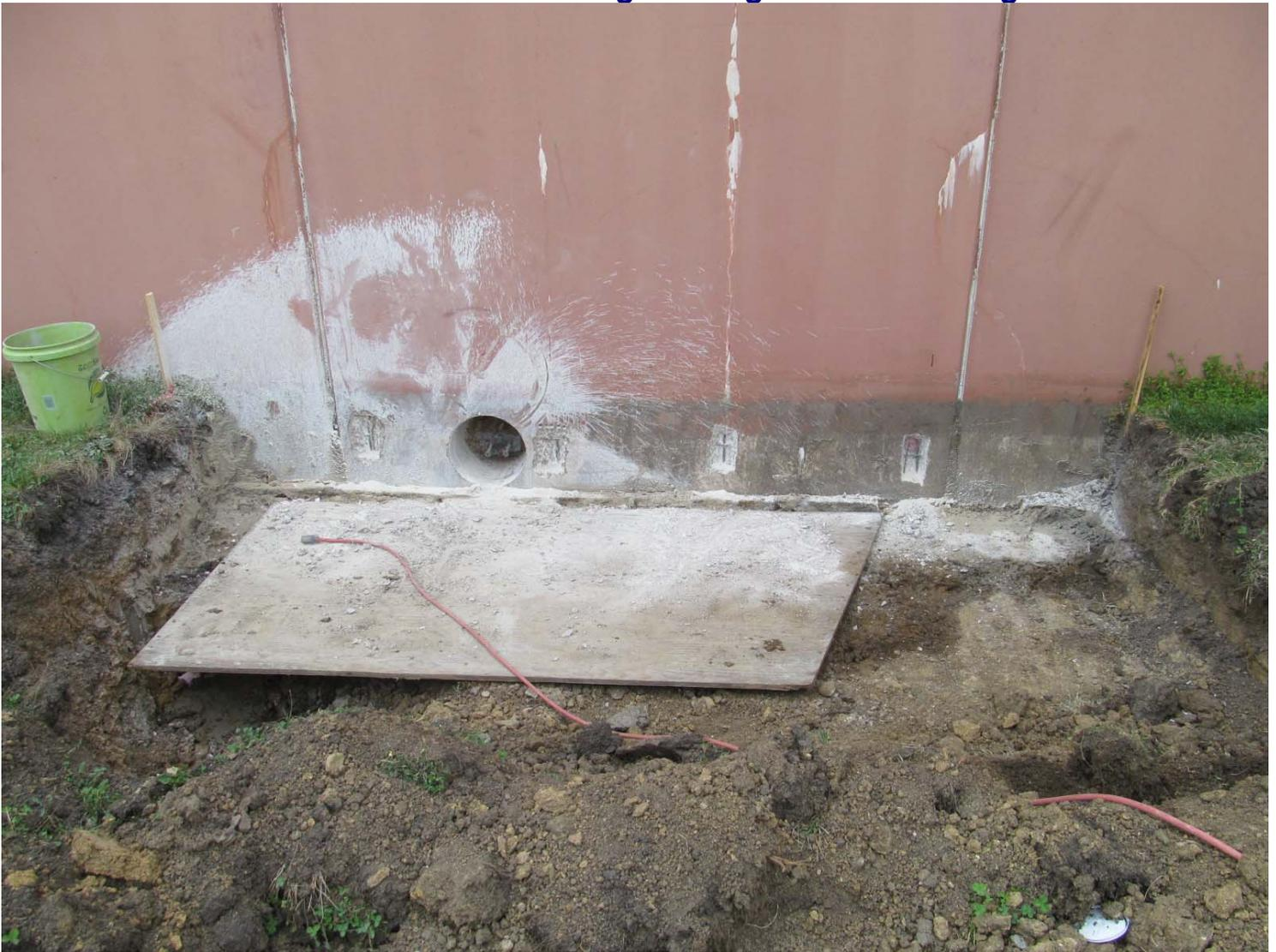
**Photograph #4: Close-up of Photograph #1 showing Vertical Cracking The Wall Panel was cored at the Base Connection, and the Prestressing Strands were exposed. The Base Connection was buried in moist sand and exhibited surface rust. One strand exhibited surface rust. The other three strands were in good condition.**
