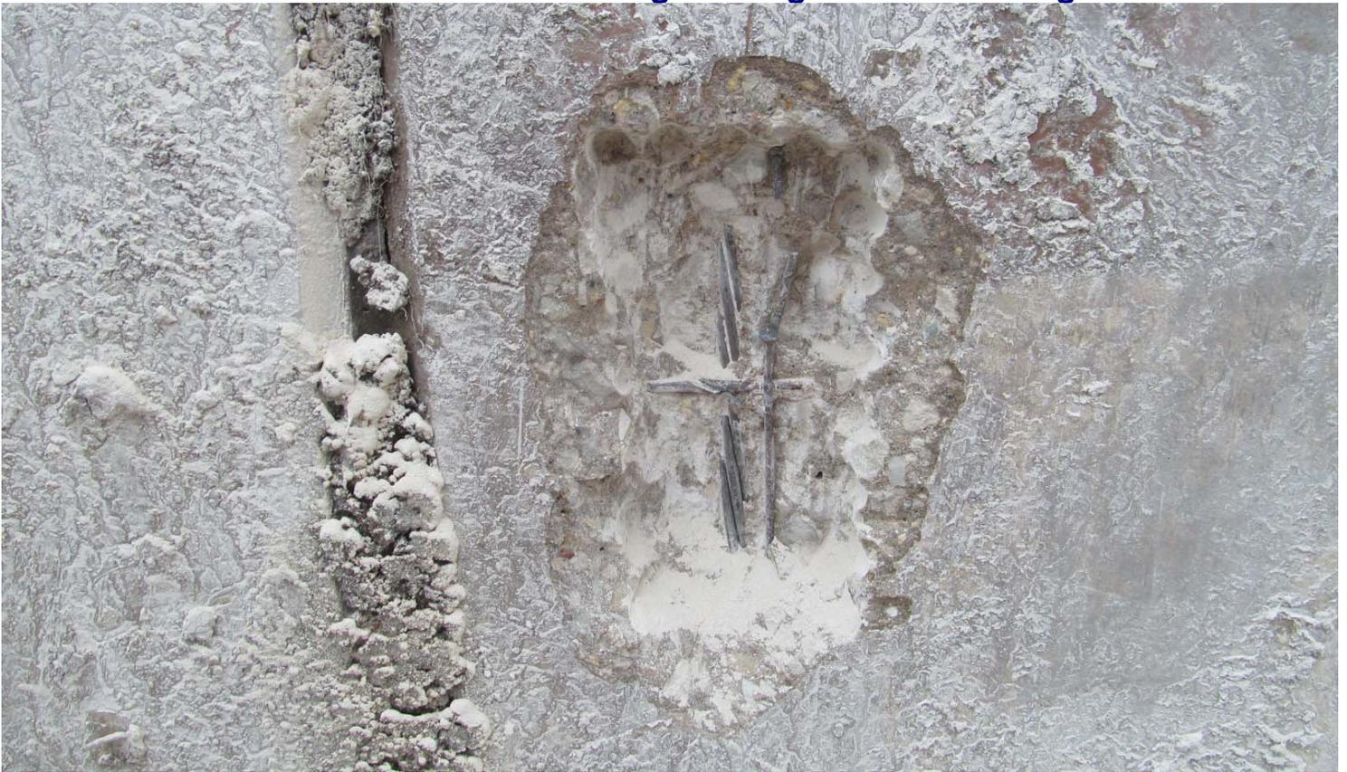
**Photograph #6:** The strand on the left side of the panel was corrosion free.
