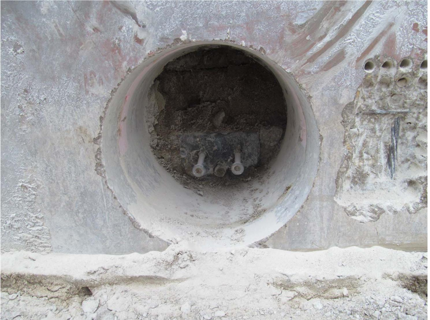
**Photograph #5: The Wall Panel Base connection exhibited surface corrosion. The steel connection is buried in sand below the floor slab. The sand was moist. The adjacent prestressing strand was corrosion free. The wall panel cracking does not extend to the bottom.**
