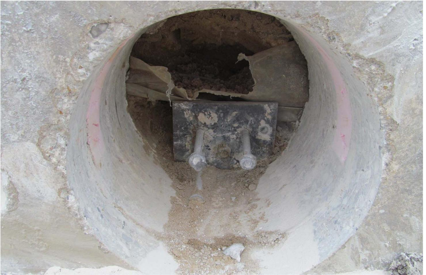
**Photograph #10: The Wall Panel Base connection exhibited surface corrosion on the buried face. The steel connection is buried in moist sand below the floor.**
