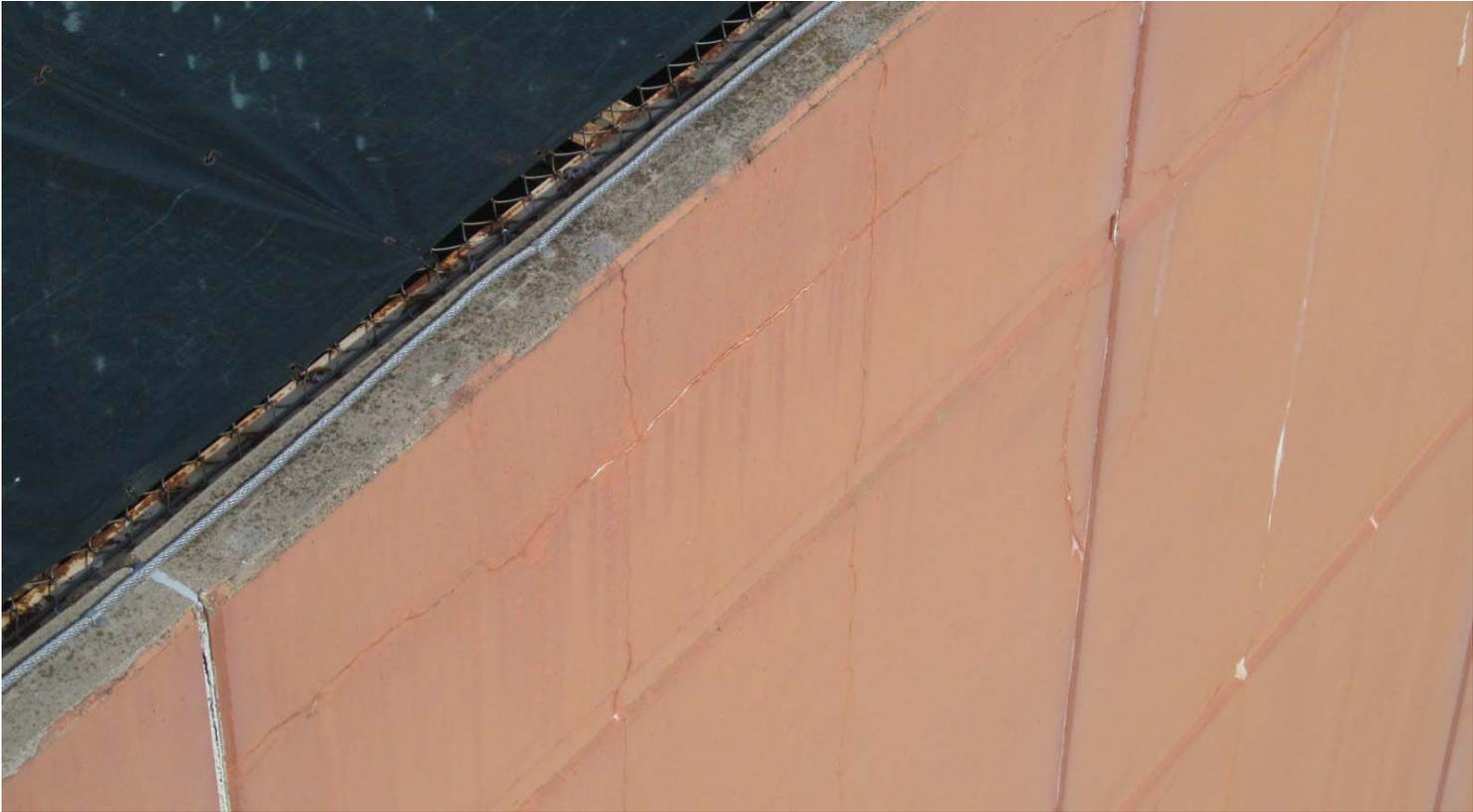
**Photograph #24: East Exercise Yard Wall Cracking**
