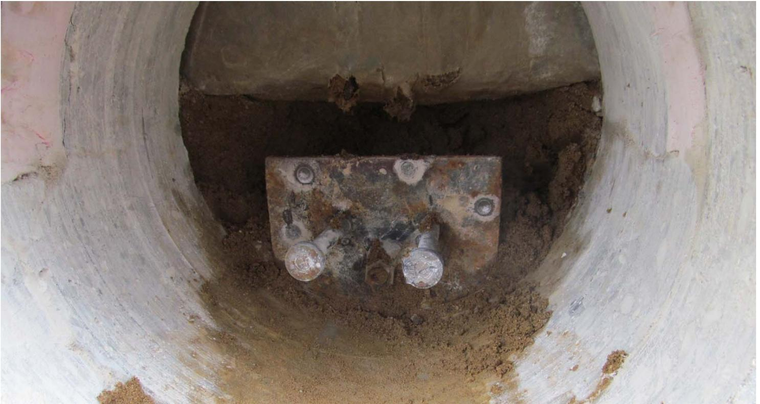
**Photograph #16: The Wall Panel Base connection exhibited surface corrosion on the buried face. The steel connection is buried in moist sand below the floor.**
