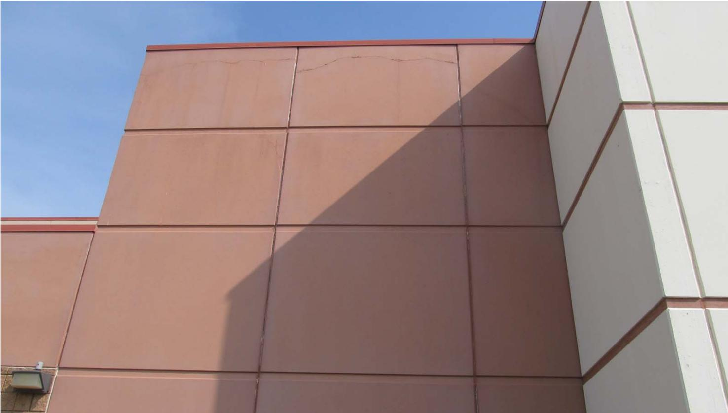
**Photograph #22: Cracking at the top of a South Wall Panel**
