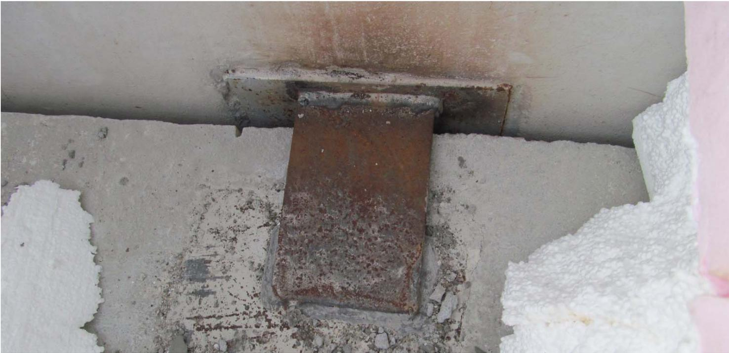
**Photograph #29: Rust on roof plank / wall panel connection, SW Corner**
