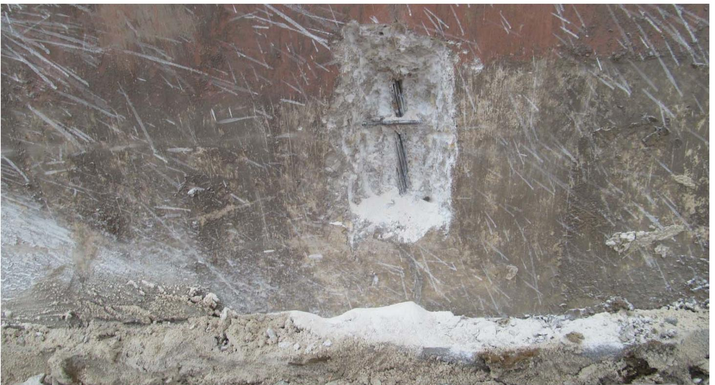
**Photograph #7:** The right-center strand exhibited surface corrosion.
