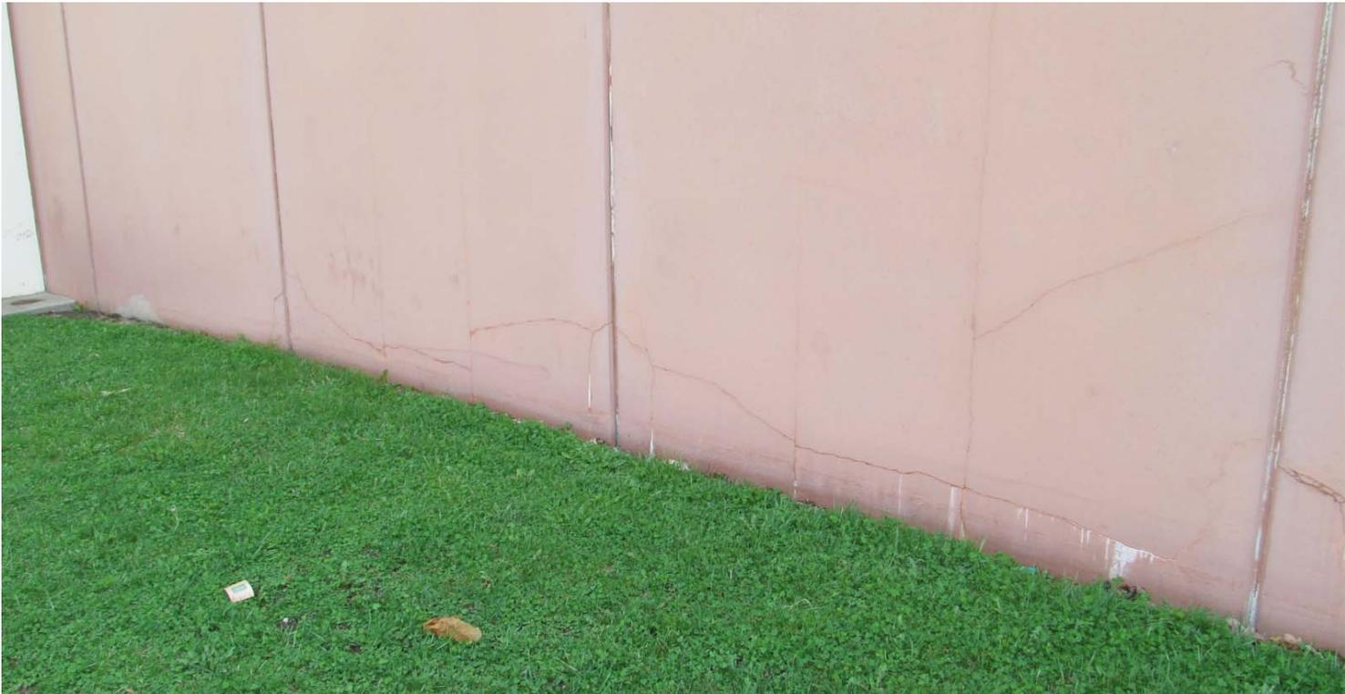
**Photograph #23: Cracking at the ground line of a West Wall Panel**
