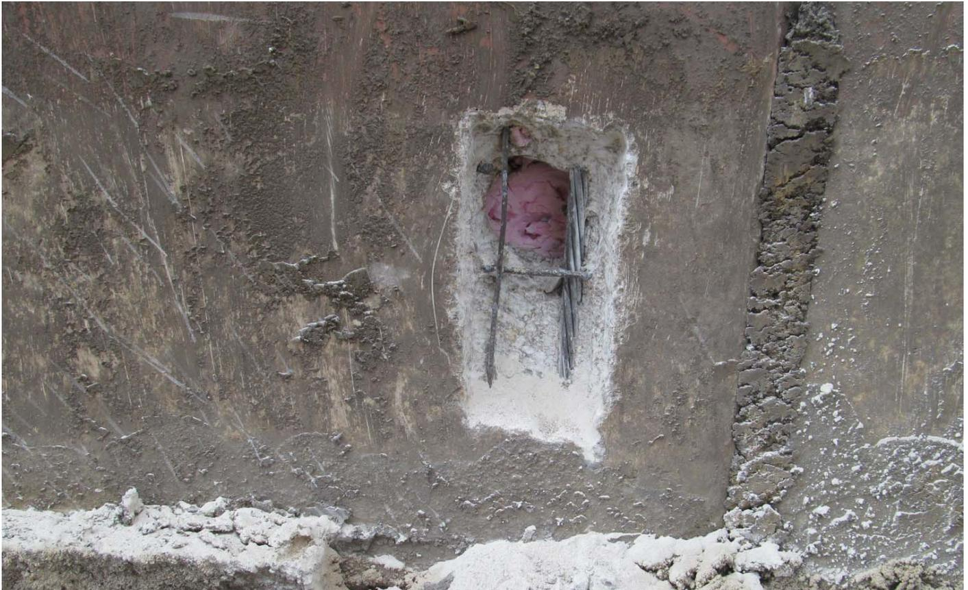
**Photograph #8: The strand on the right side of the panel was corrosion free.**
