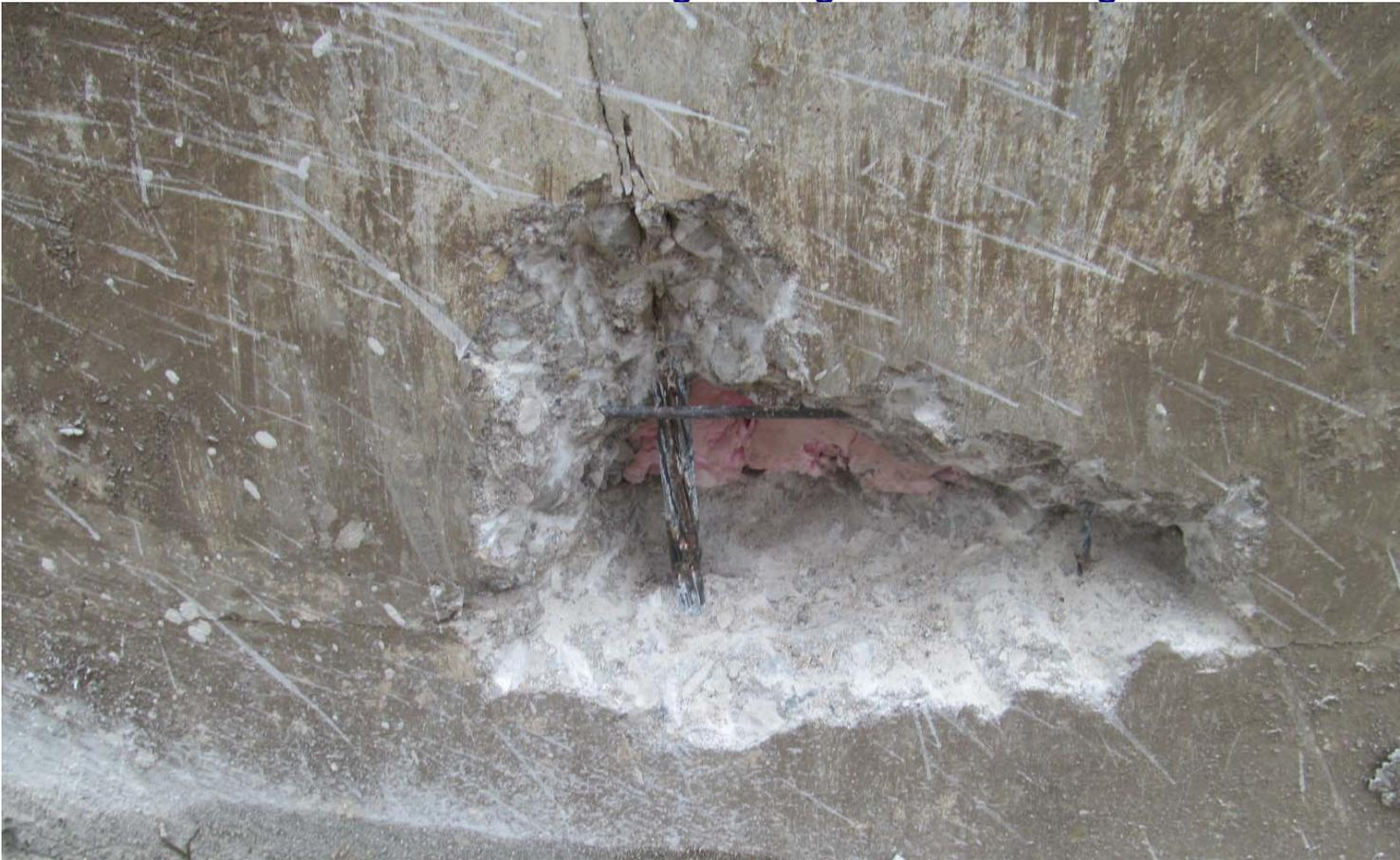
**Photograph #19: The right-center strand exhibited surface corrosion.**
