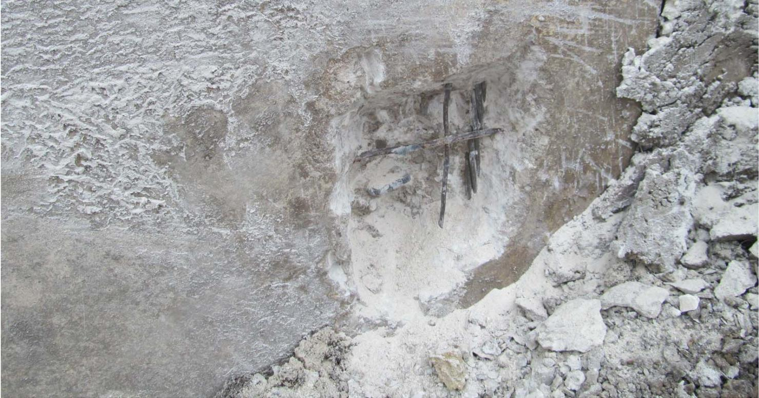
**Photograph #14: The strand on the right side of the panel was corrosion free.**
