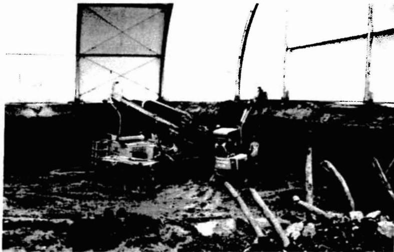
Inside the tent, specially trained workers remove source material and contaminated soil. The material is hauled away in covered trucks. Clean fill is then placed in the excavated area. Photo taken at the Ameren Illinois Utilities MGP remediation in Jacksonville.
