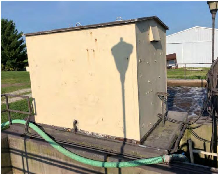
Figure 2-12 Chlorine Contact Tank with Chlorine Building
