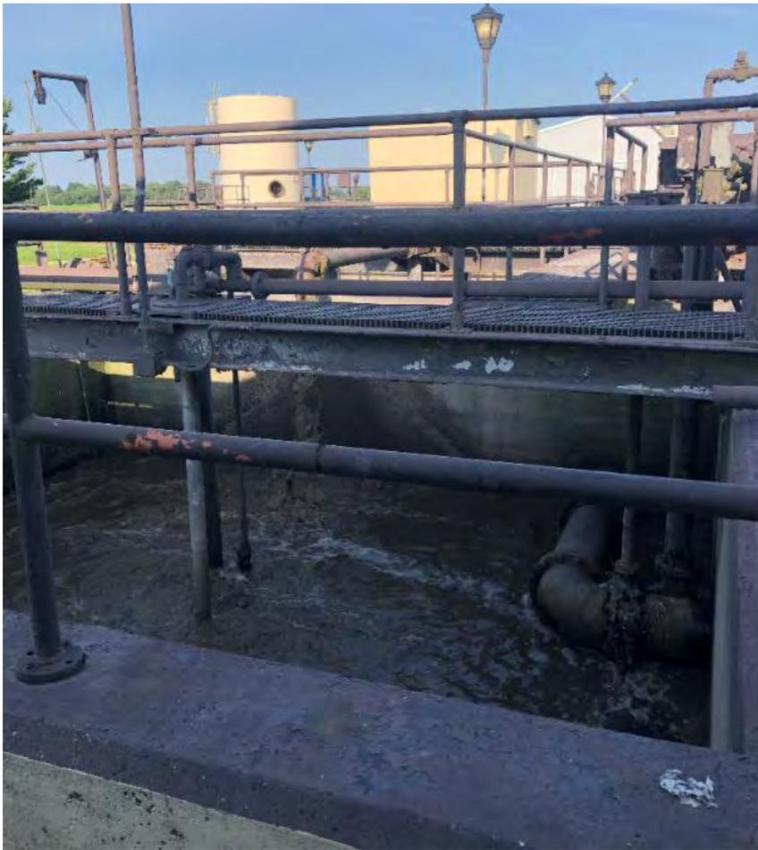
Figure 2-13 Aerobic Digester
