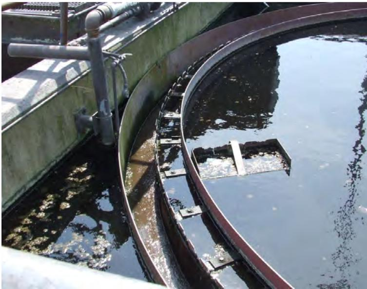
Figure 2-11 Final Clarifier Effluent Weir
