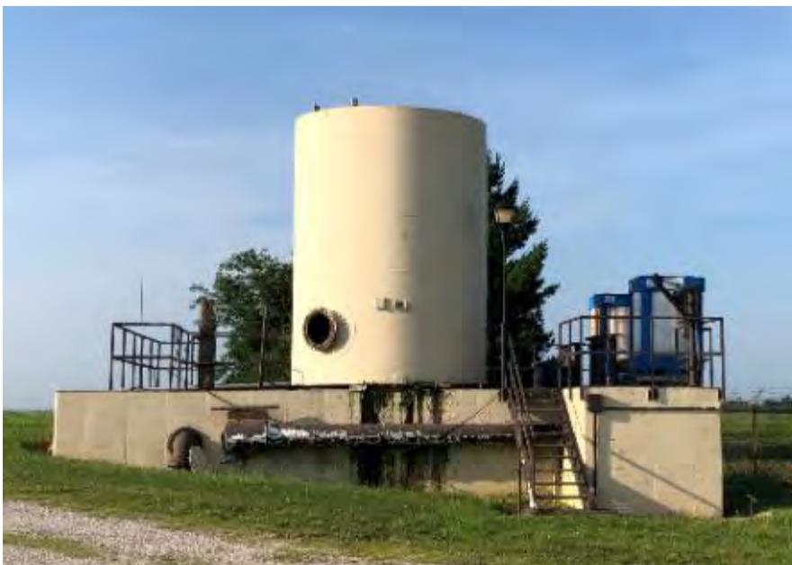
Figure 2-7 Primary Clarifier and Roughing Filter
