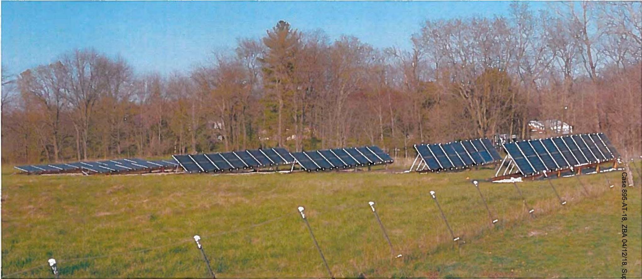
**Panels are retilted 4 times/year, at 12, 38, 65° and 38° (summer, fall, winter and spring), resulting in 13% greater production than installer estimated values for a constant 30° tilt ground mount and 33% greater than for a 14° tilt roof mount.**
