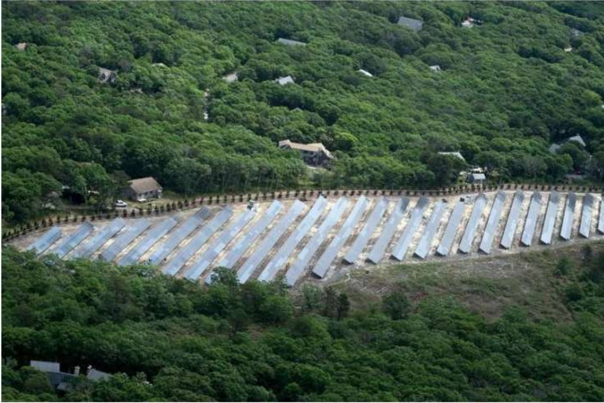
Solar panel array occupies 5.8 acres.
