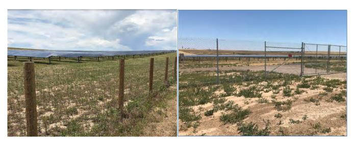
Photo 2. Fencing Options including agricultural style fencing (left) or chain link (right).
