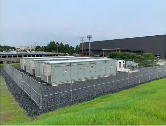
This utility-scale ESS in Vermont is using li-ion batteries to provide peak reduction and frequency regulation services. Photo courtesy of WEG. Source: Energy Storage Systems based on the IBC, IFC, IRC, and NEC, International Code Council, January 2022
